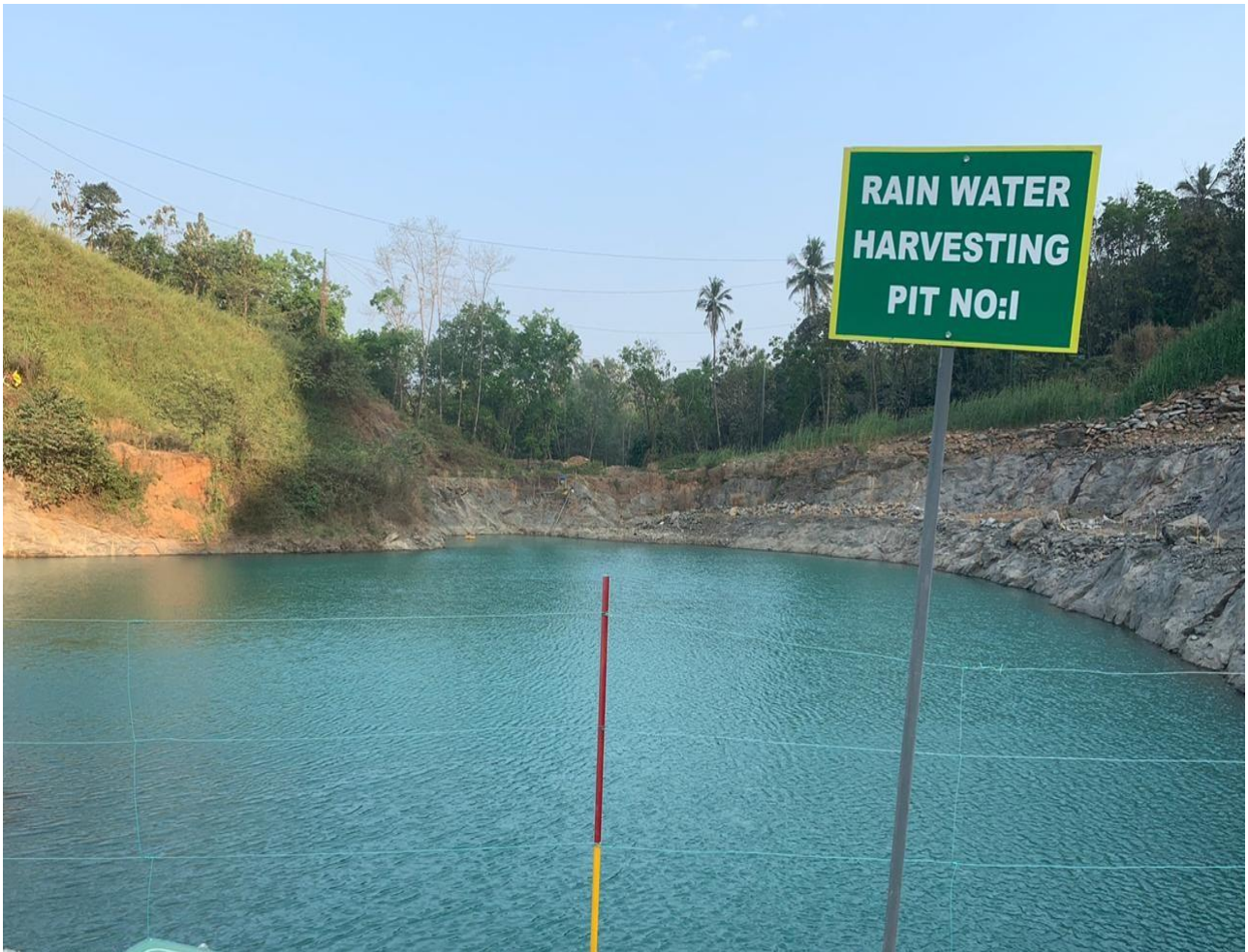
Fig 1 Rainwater Harvesting Pond
