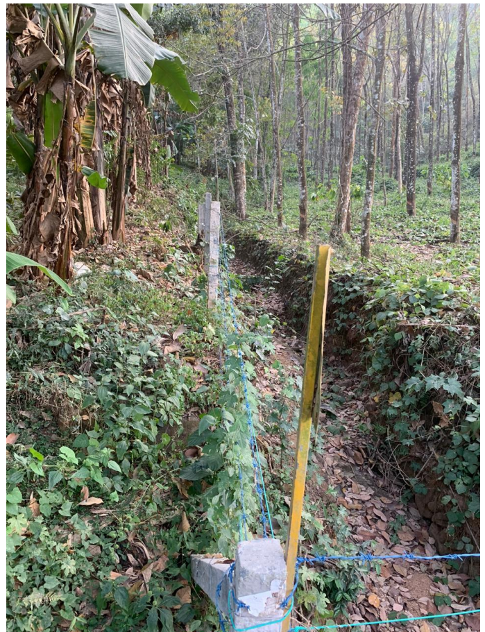
Fig 4.2 Barbed wire fencing
