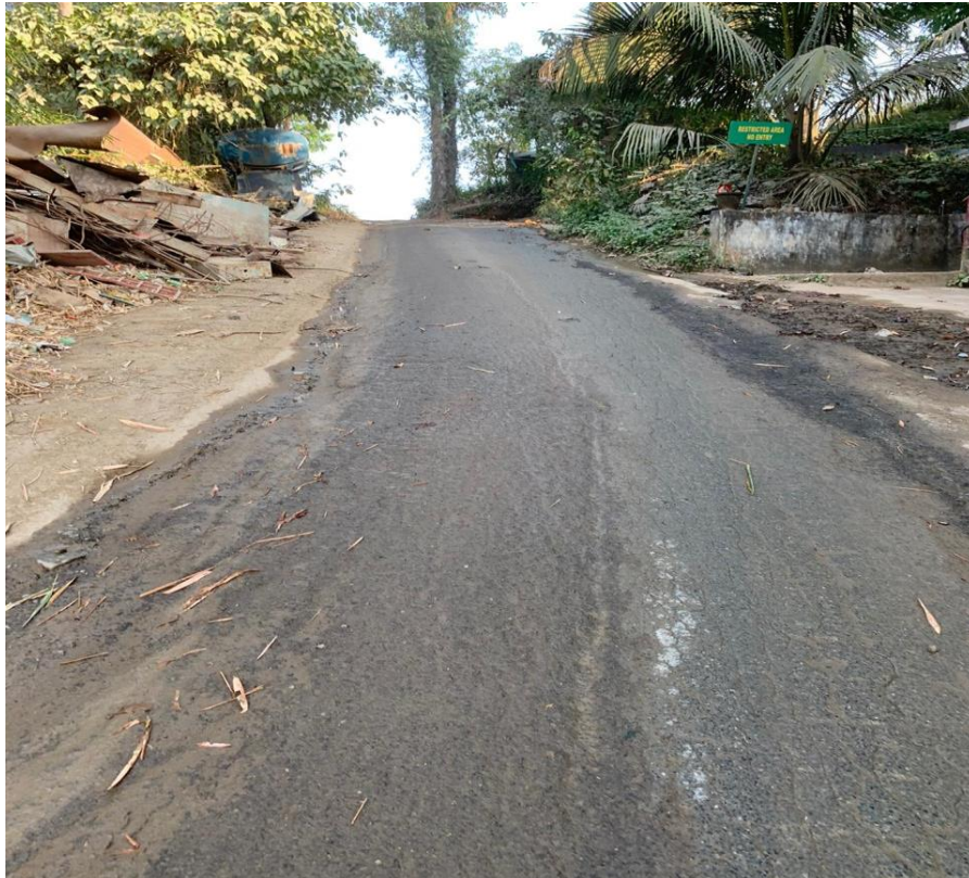
Fig 6. Tarred access road
