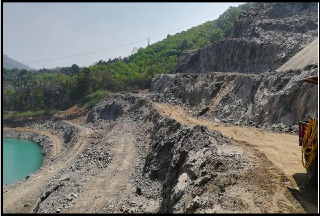
Bench system in the quarry
