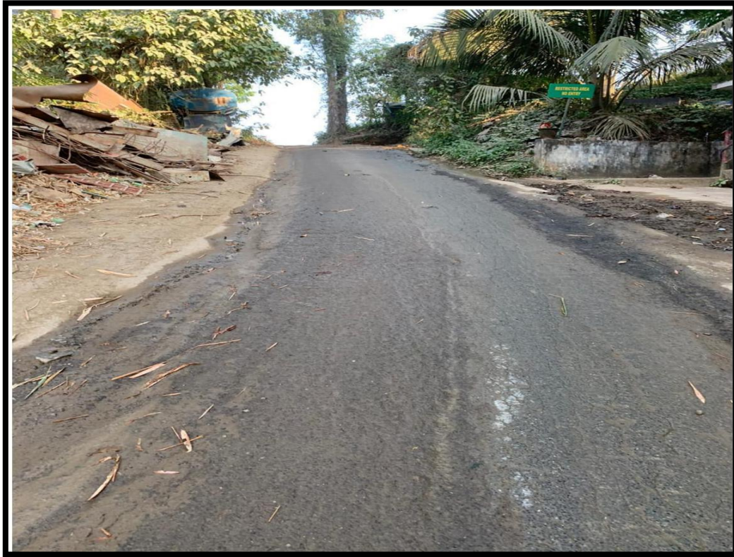
Tarred road to the quarry
