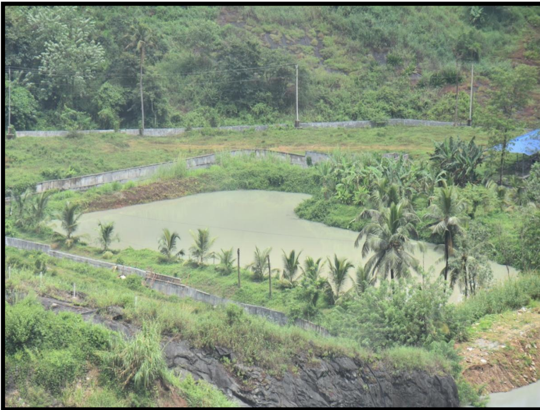
Rain water harvesting pond
