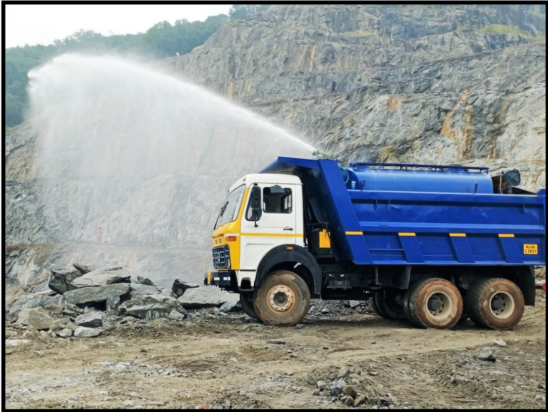
Water sprinkling before blasting and loading
