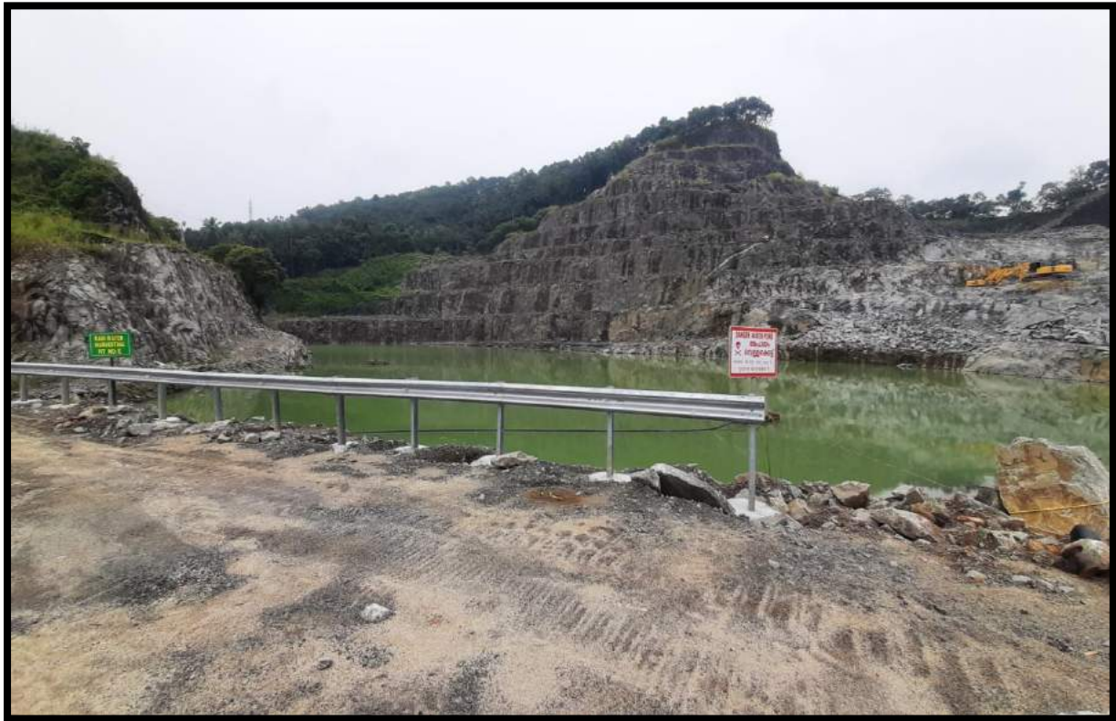
Fencing around Rain water harvest pond
