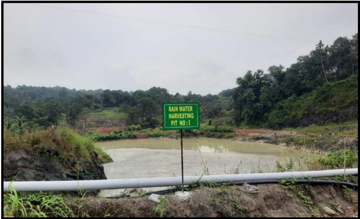
Rain water harvesting pond
