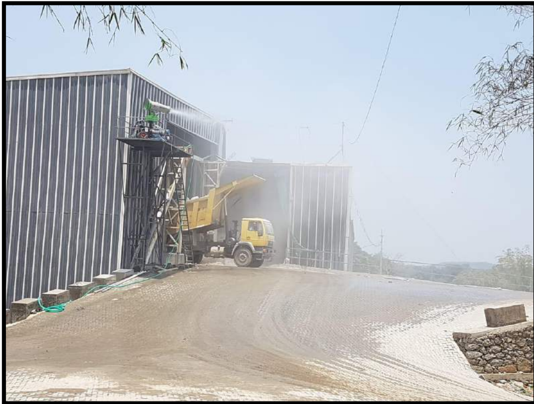
Water spraying at unloading point (hopper) of crusher.
