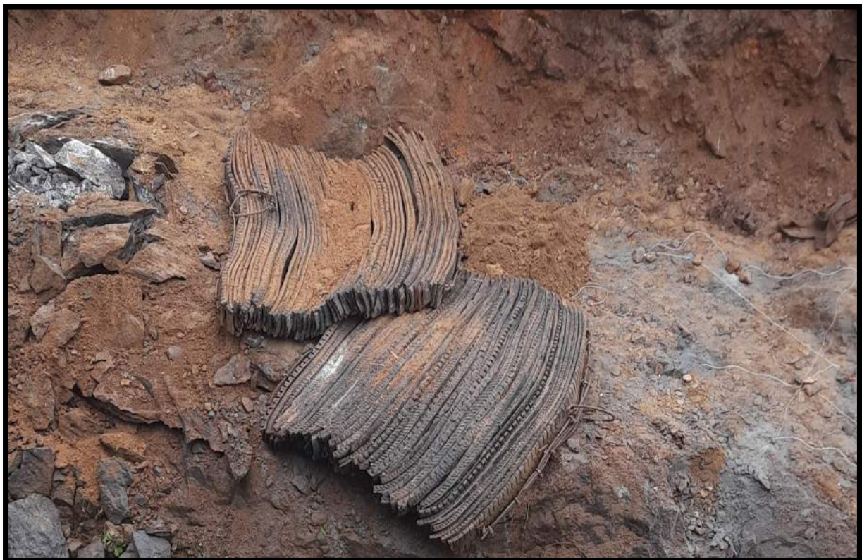
Blasting mats in use
