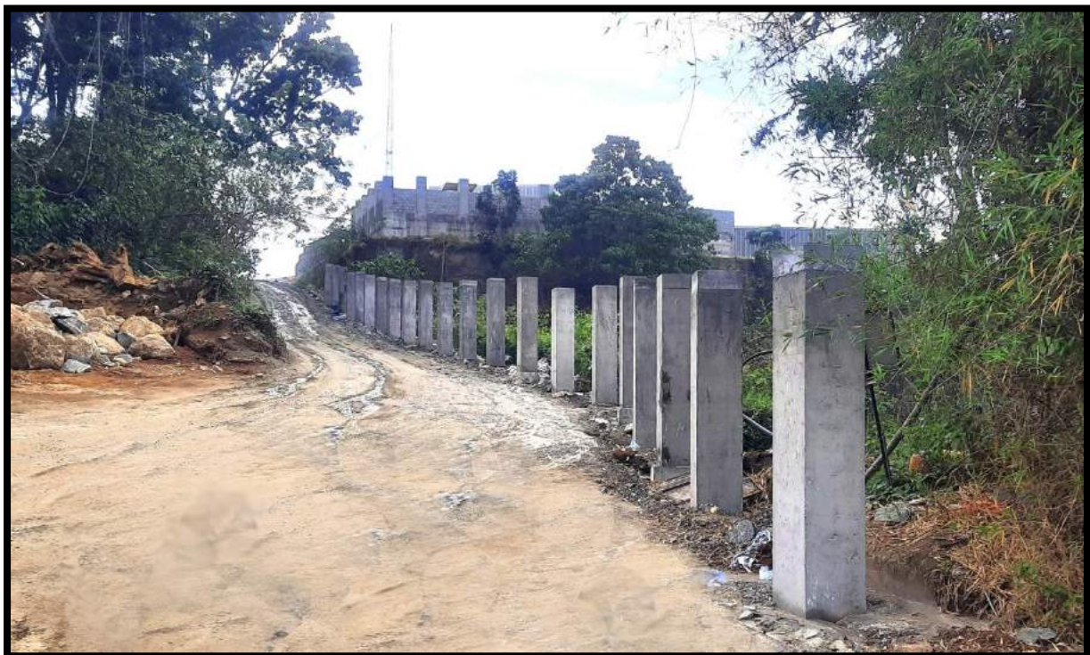
Protection wall construction
