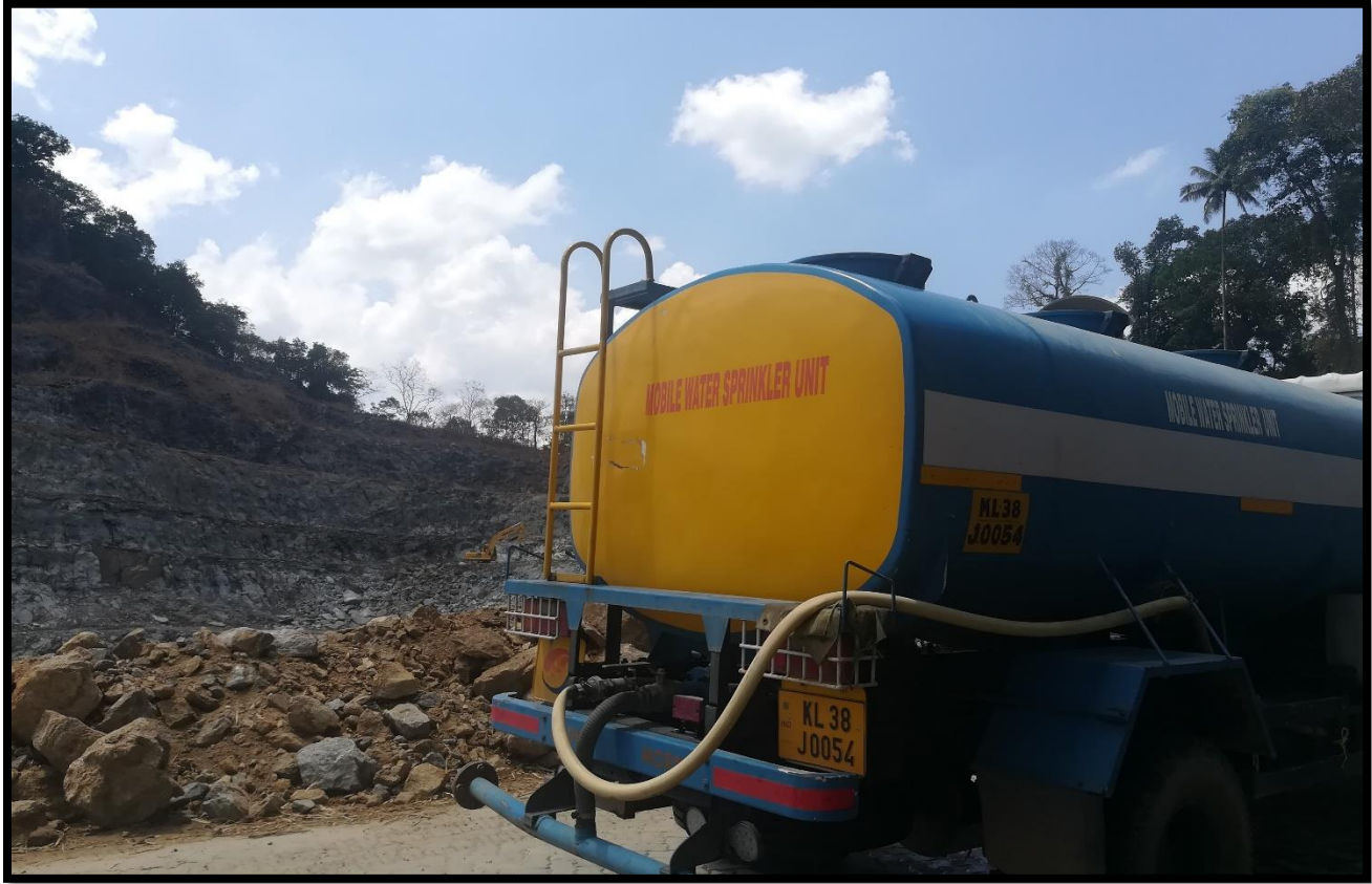
Water Sprinkler Unit
