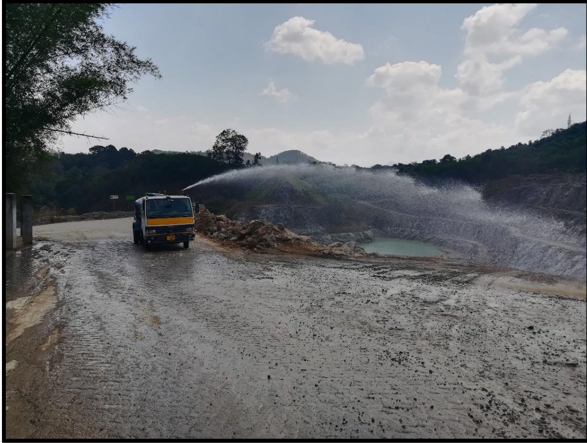
Water Sprinkling done on Necessary Roads
