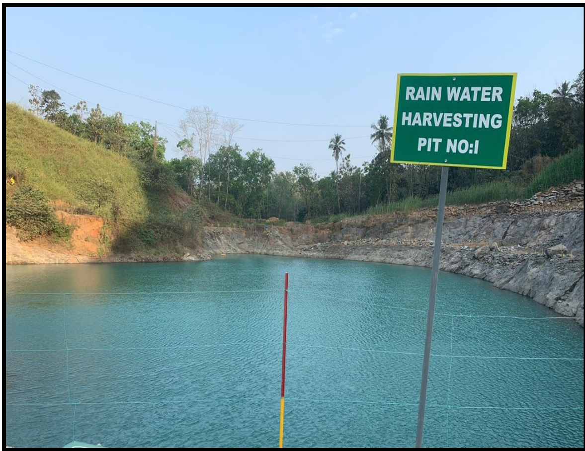
Rain Water Harvesting Pond 1
