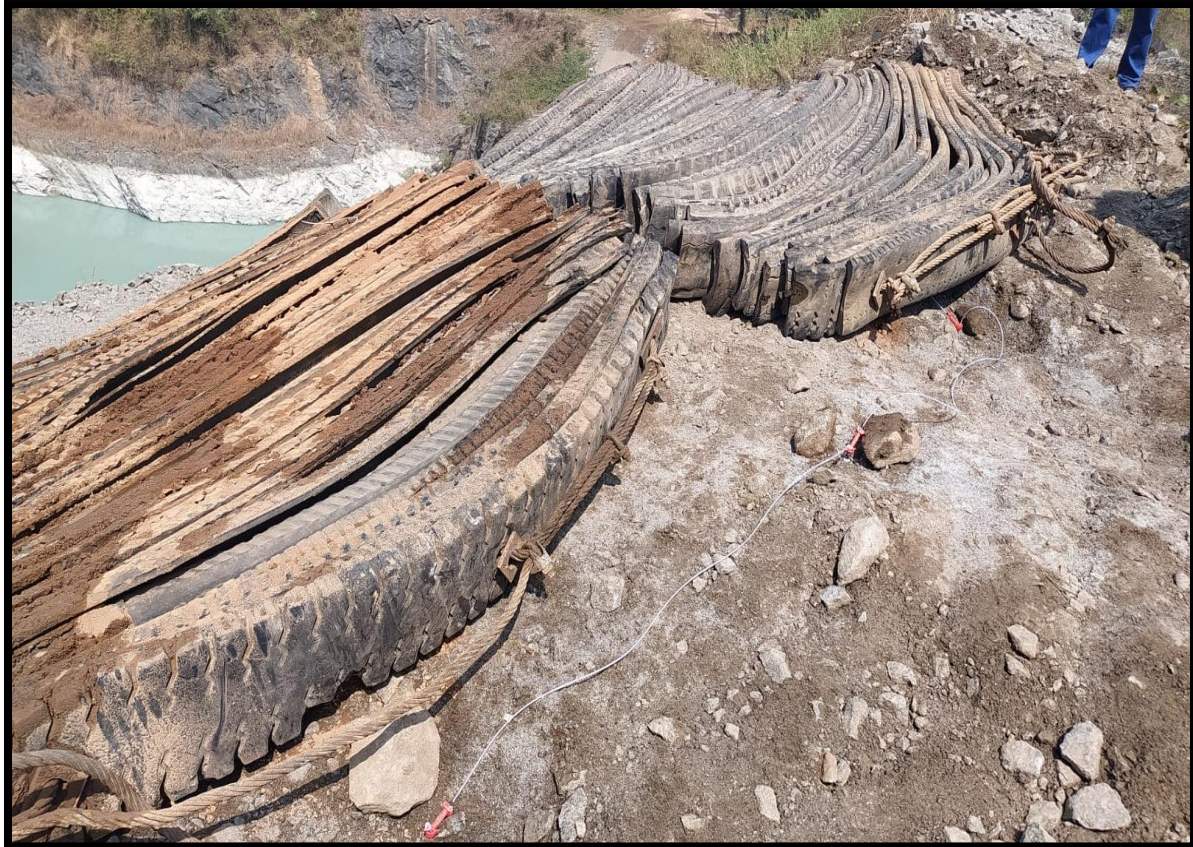
Blasting Mats on Top of Charged Holes
