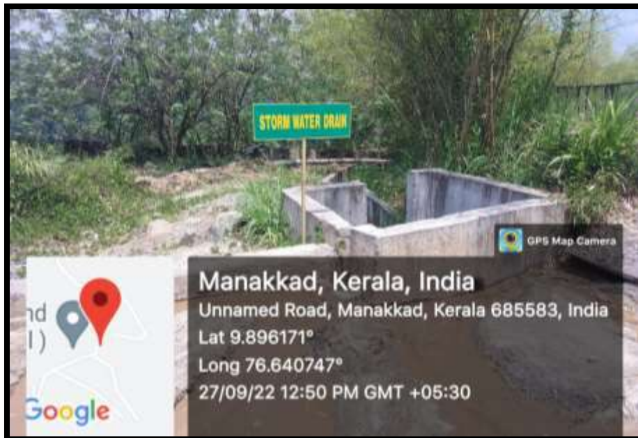
Storm Water Drain
