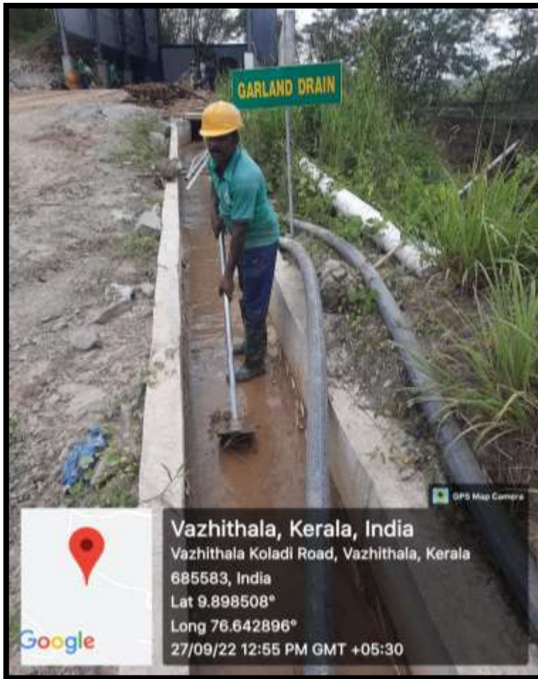
Garland Drain Cleaning work
