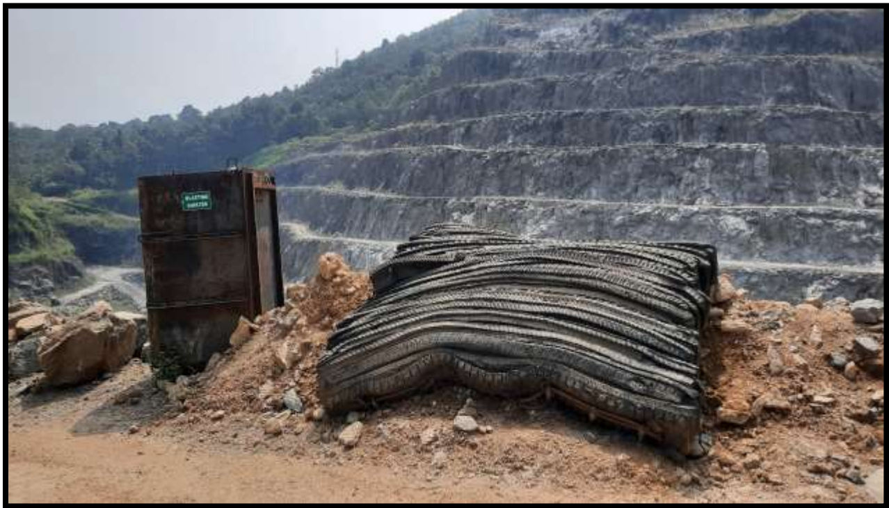
Blasting Shelter & Blasting Mats
