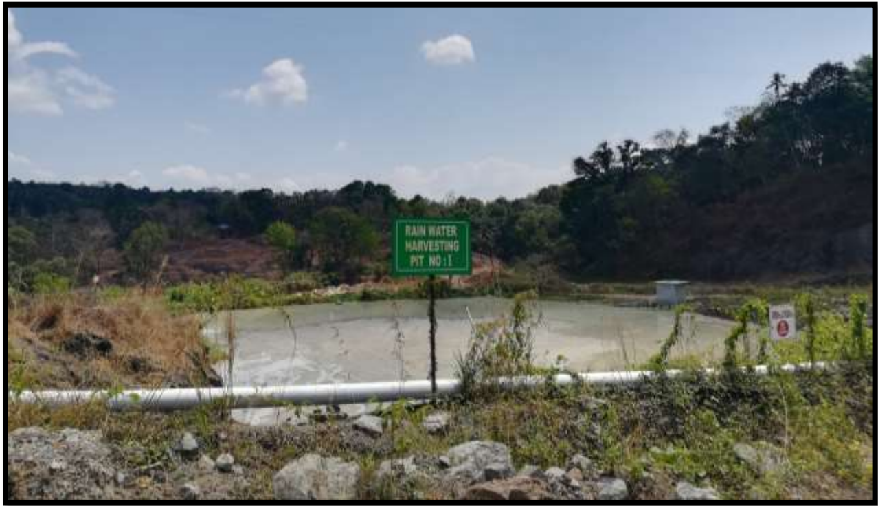
Rain Water Harvesting Pit-I
