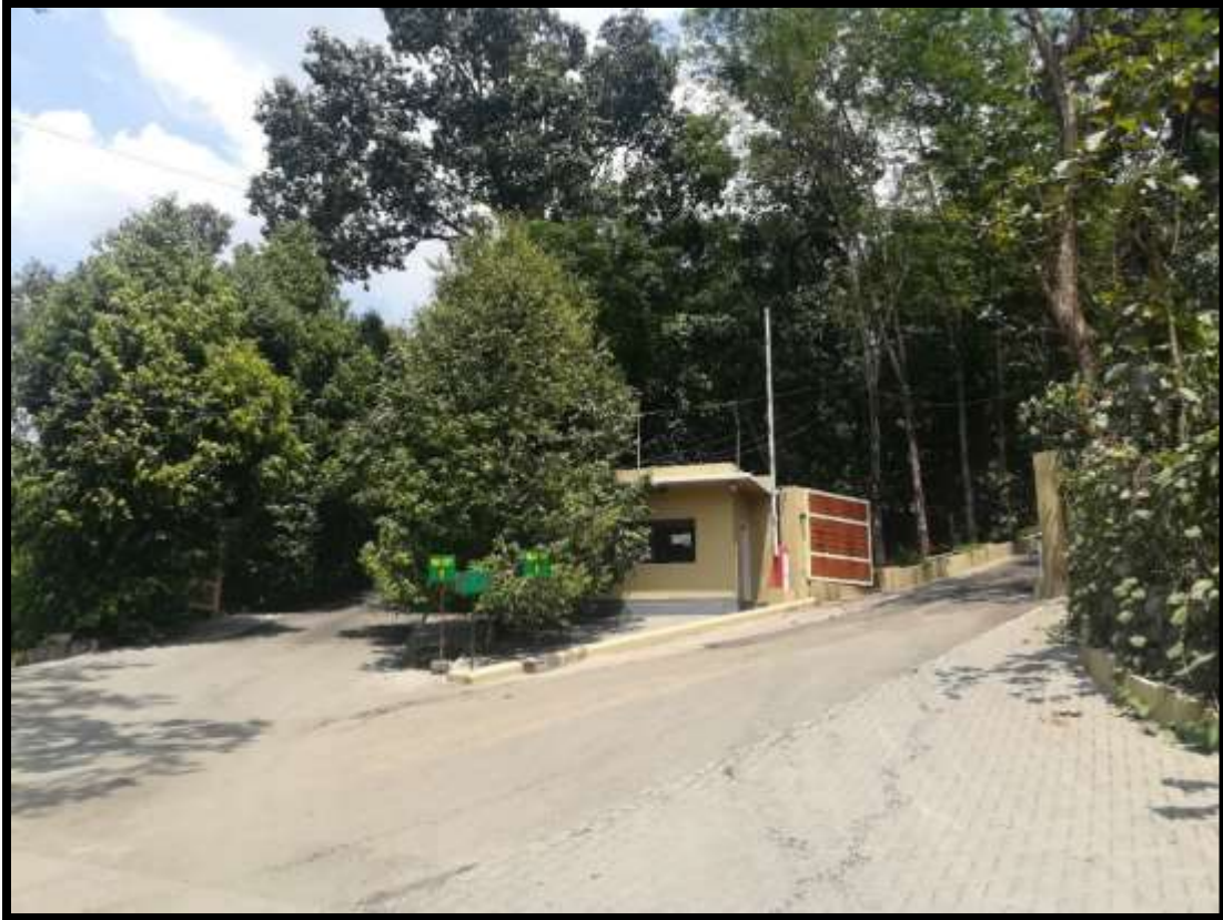
Tarred Access Road
