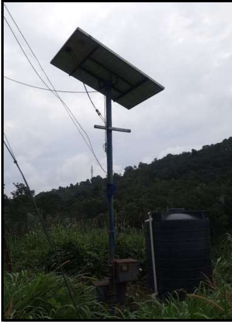
Solar Light installed at the site
