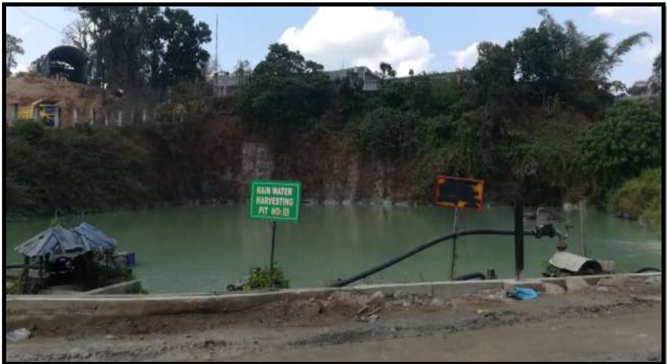
Rain Water Harvesting Pit-III
