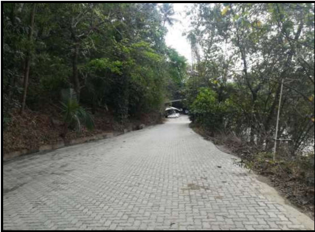
Tiled Quarry Road
