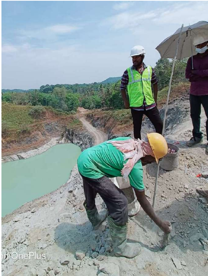
Fig 9: Stemming of Blast Holes
