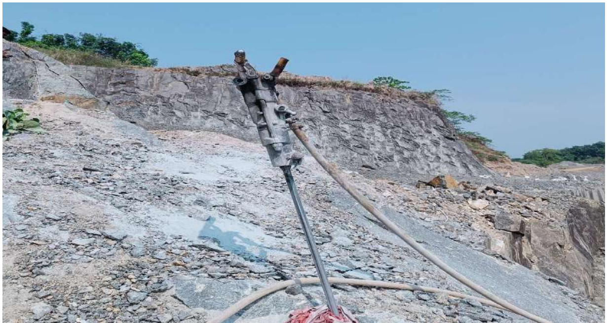
Fig 5: Drilling of Blast Holes using Jack Hammer
