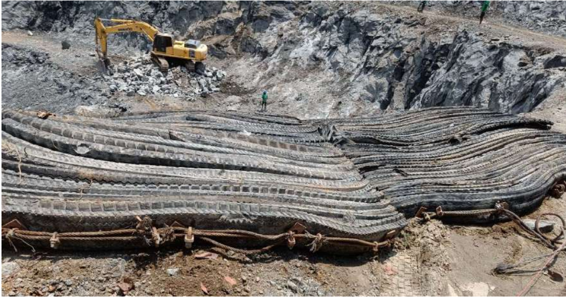
Fig 11: Muffling arrangements to control the Fly rocks
