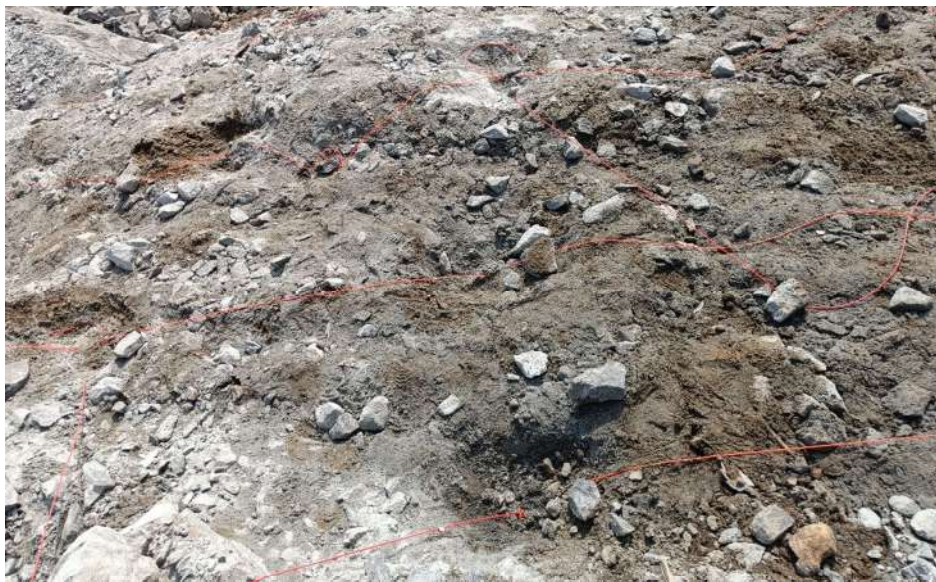
Fig 10: Charged Holes
