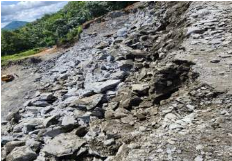
Fig 13: Fragmented Rock after Blasting
