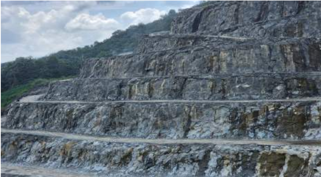
Fig 7: A Close view of the Bench Face
