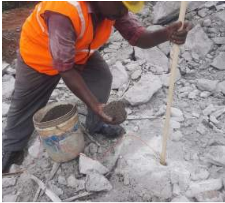
Fig 10: Stemming of Blast holes
