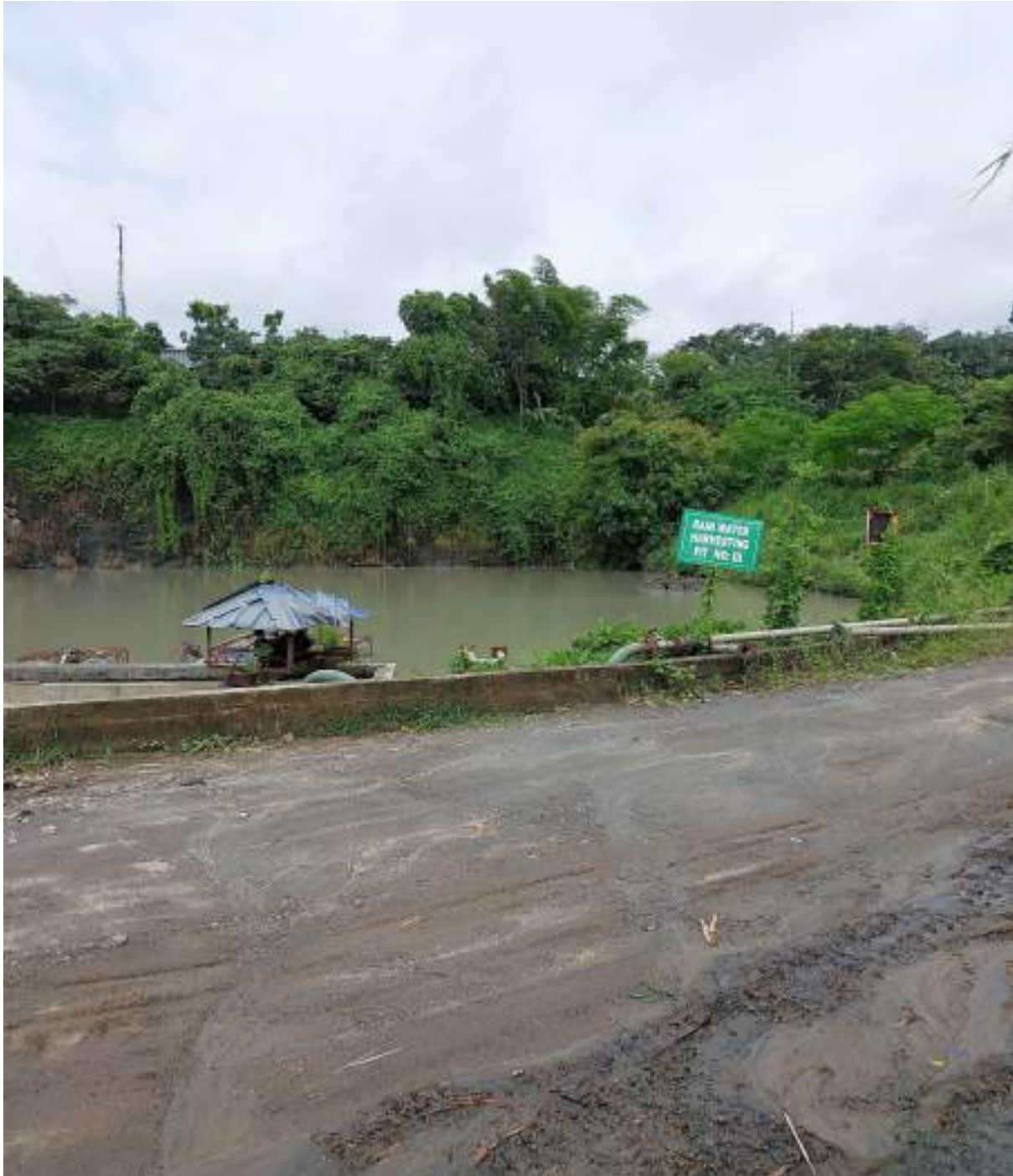
Rainwater Harvesting Pond
