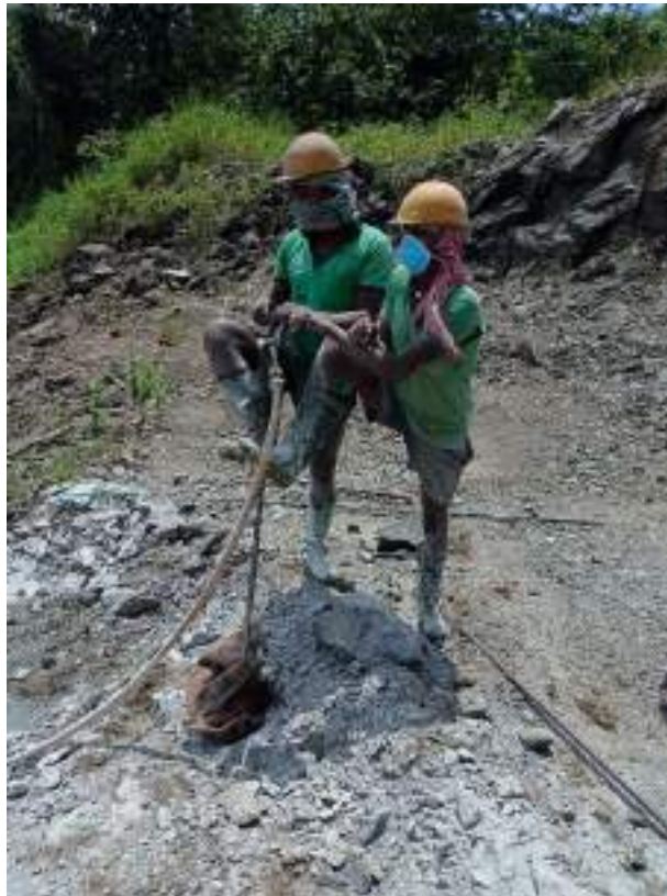
Fig 6: Drilling of Blast Holes using Jack Hammer
