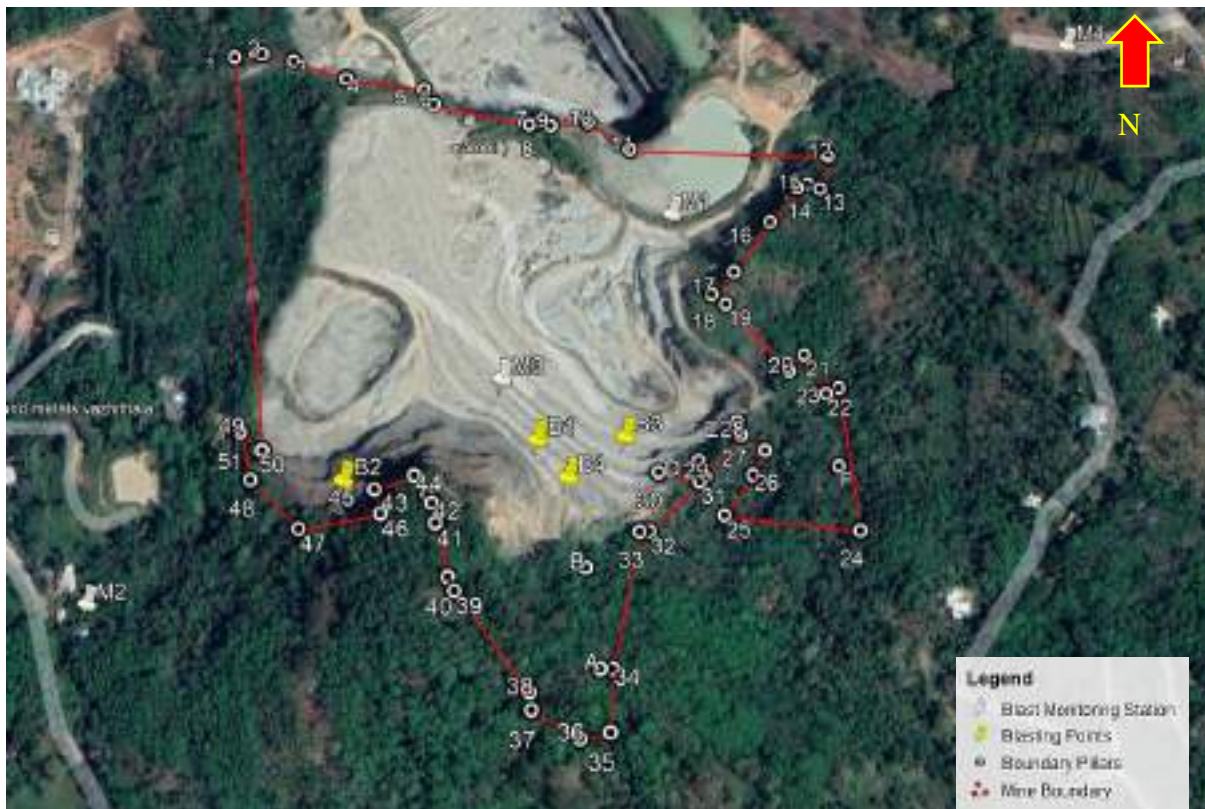
Fig 4: Google Earth Image of the Mine showing Blasting Locations & Monitoring Points
