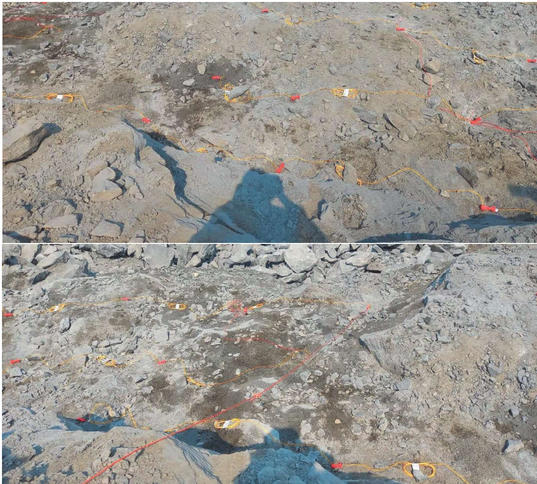
Fig 11: Charged Holes
