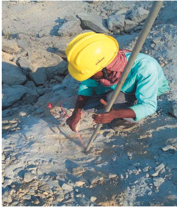
Fig 10: Stemming of Blast holes
